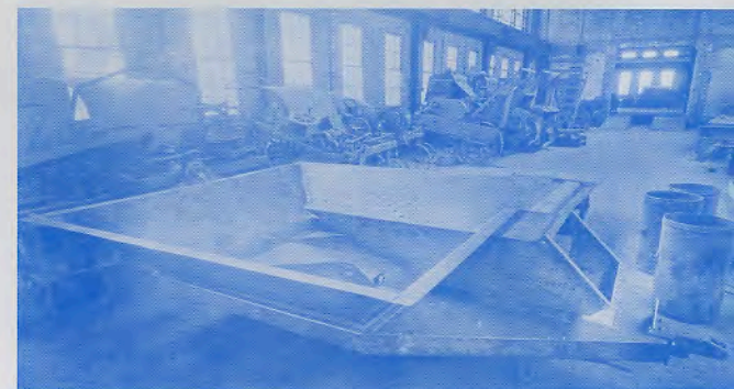
The assembly floor in January 1927. Sandcutters in various stages of production are shown at left.
